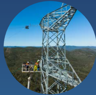
Electricity into existing 220kV power line
